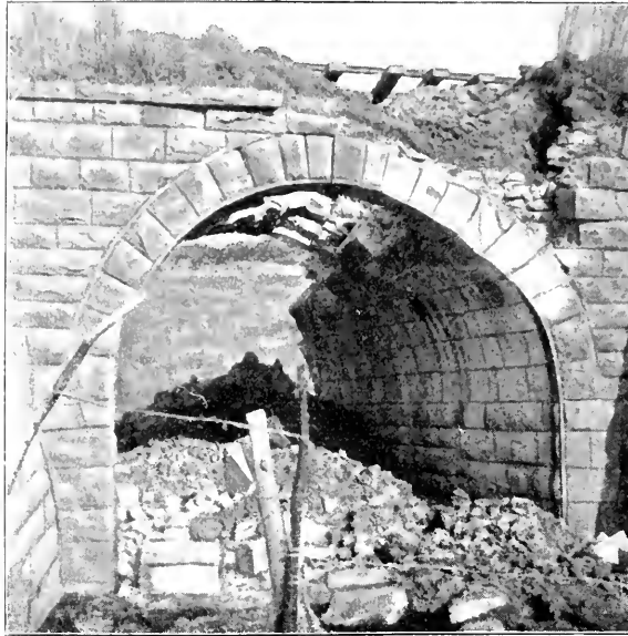
VIADUCT IN THE BIGGARSBERG (Natal), WRECKED WITH DYNAMITE BY THE BOERS.
